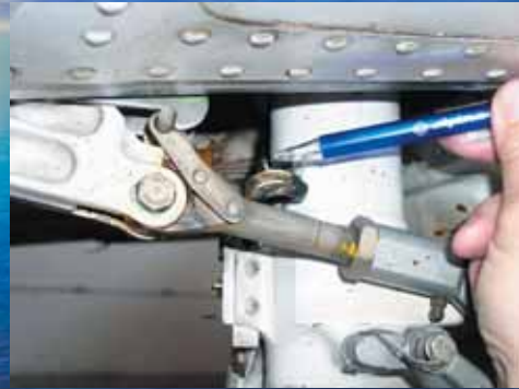
Cause of the PA-44 accident: micro switch failure
